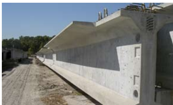
Vapor cured bulb-T members await transport and final installation on Atlanta Hartsfield's fifth runway project.
