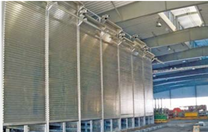
Automatic insulated roller-shutter doors provide the benefit of insulation for conden- sation reduction.
